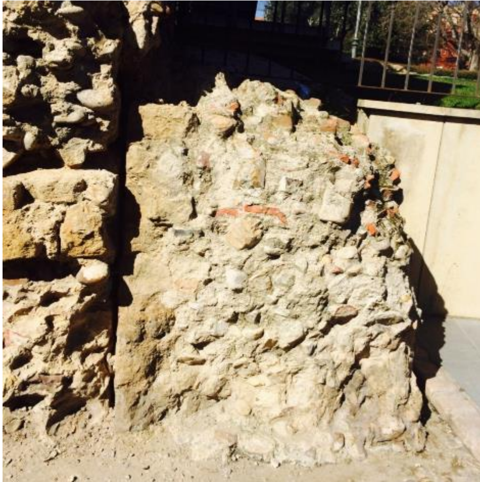
Fig. 59 Photograph of Calle Ruiz de Salazar. Roman wall with large fragments of tegulae in the concrete filling. On the left, attached to its outer ashlar face, the wall of cubos .
