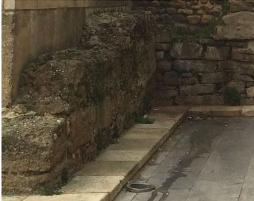
Fig. 75. Detail photograph of the connection point of the flanking tower of the so called porta principalis sinistra with the walls of the Roman fortified precinct and the later wall of cubos . Detail of the construction systems of the tower—with non-padded sandstone ashlar and shod with rubble—, and the lower part of the medieval wall of cubos , made of ordinary squared quartzite stonework.
