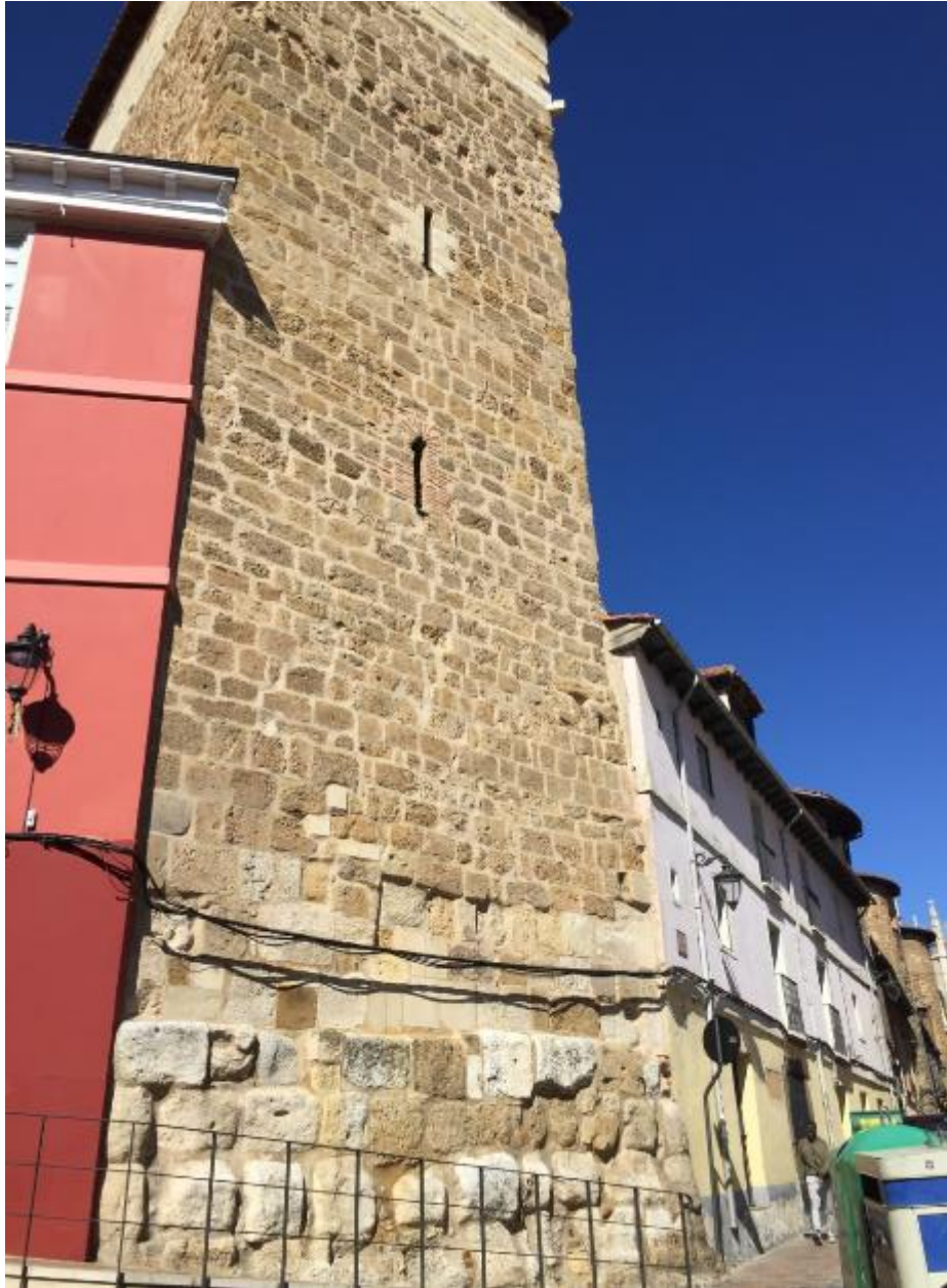
Fig. 71. Torreón de los Ponce (in the southeast corner of the Roman camp of León), which preserves the foundation or base of large padded ashlars.
