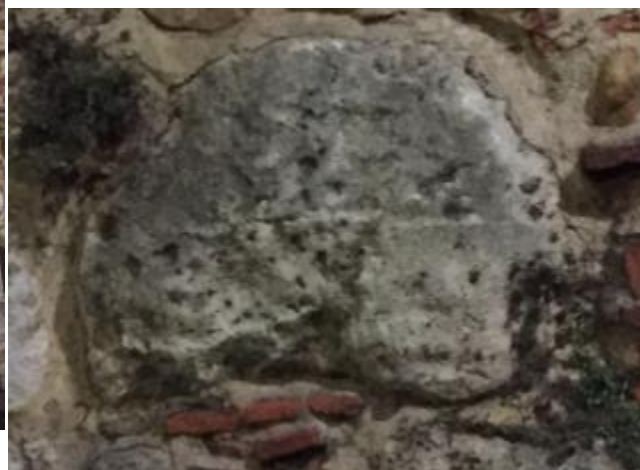
Figs. 39 and 40. Tower of the medieval wall of León built with reused Roman funerary cuppae . Detail of the cuppa .
