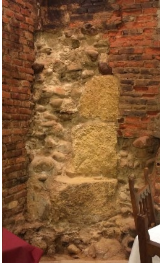
Fig. 70. Commercial premises in Calle La Rúa, back wall: it borders the wall in Conde Rebolledo. Corner ashlars possibly corresponding to the Roman tower at the SW corner of the Roman camp in León.
