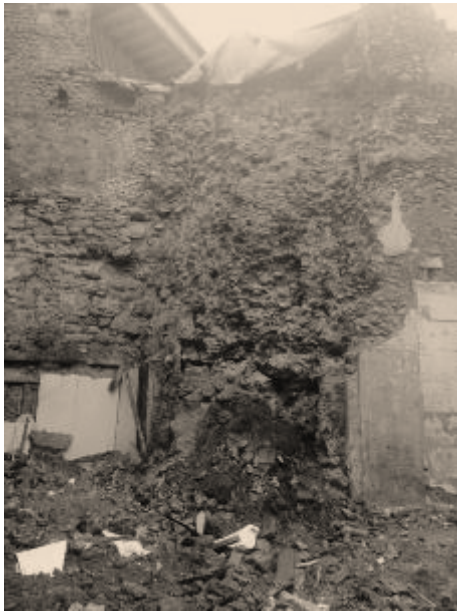
Figs. 108 and 109. State of the cubo at the southwest corner of the medieval wall after it collapsed in 2017: we can observe the filling layer of the cubo overlapping the medieval facing of the wall.
