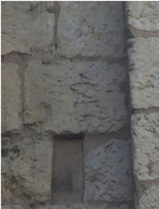
Fig. 9. Detailed photograph of ashlar with VI mark in situ on a blocked putlog hole. Tower of San Isidoro (León).
