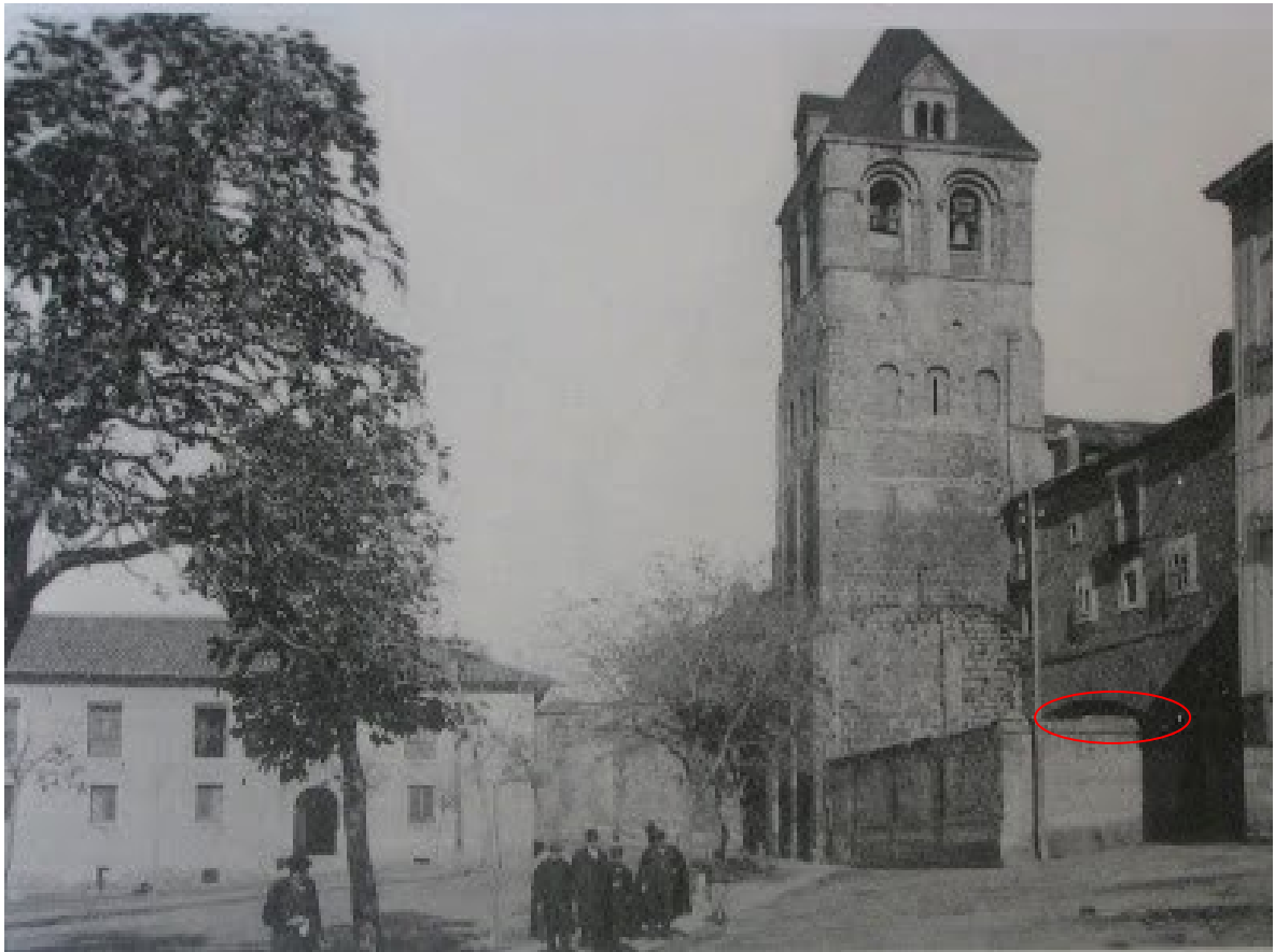
Fig. 63. Old photograph of San Isidoro Tower. To its right and almost hidden by a corner enclosure, you can see the open arch in the section of the wall of cubos on which two floors of a building were erected.
