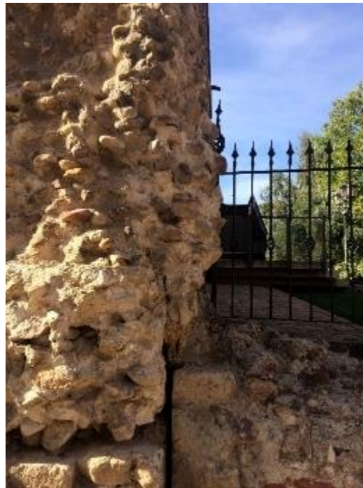
Figs. 79 and 80. Detail of breach between the two walls, the Early Imperial Roman wall and wall of cubos , in Calle Ruiz de Salazar. Above the breach, part of a layer of mortar and riverstones that proves that the small-ashlar Roman wall was already in ruins when the wall of cubos was built, and it did not serve as a support higher up.
