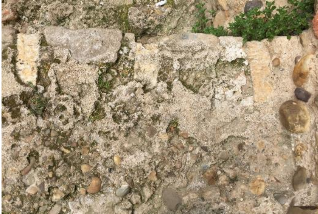
Figs. 56 and 57. Photographs of the bonding of stretchers alternating with mixed courses of header and stretcher: interfaces of the ashlar facing of the Roman wall (access to San Isidoro from Avenida Ramón y Cajal). At the top of the images, lime and stone concrete filling in the wall of cubos .
