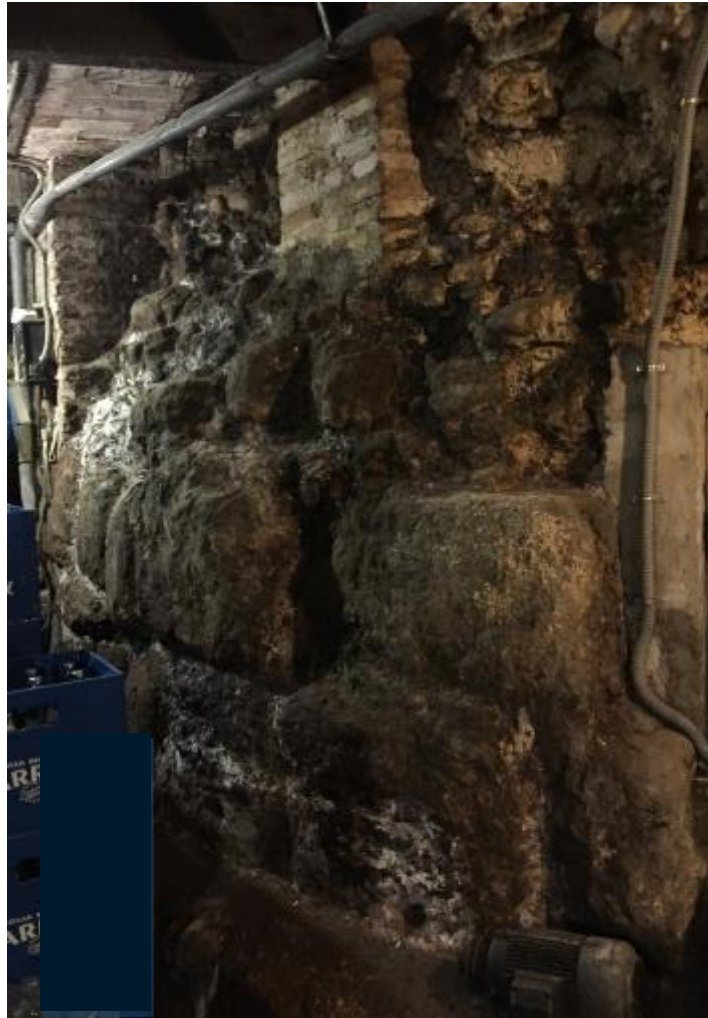
Fig. 72. Unresearched basement of a tower at the southern gate of the Roman camp in León with large padded ashlars in the wall of a cellar in Calle Azabachería.
