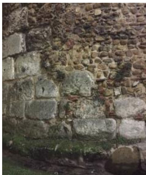
Figs. 39 and 40. Tower of the medieval wall of León built with reused Roman funerary cuppae . Detail of the cuppa .
