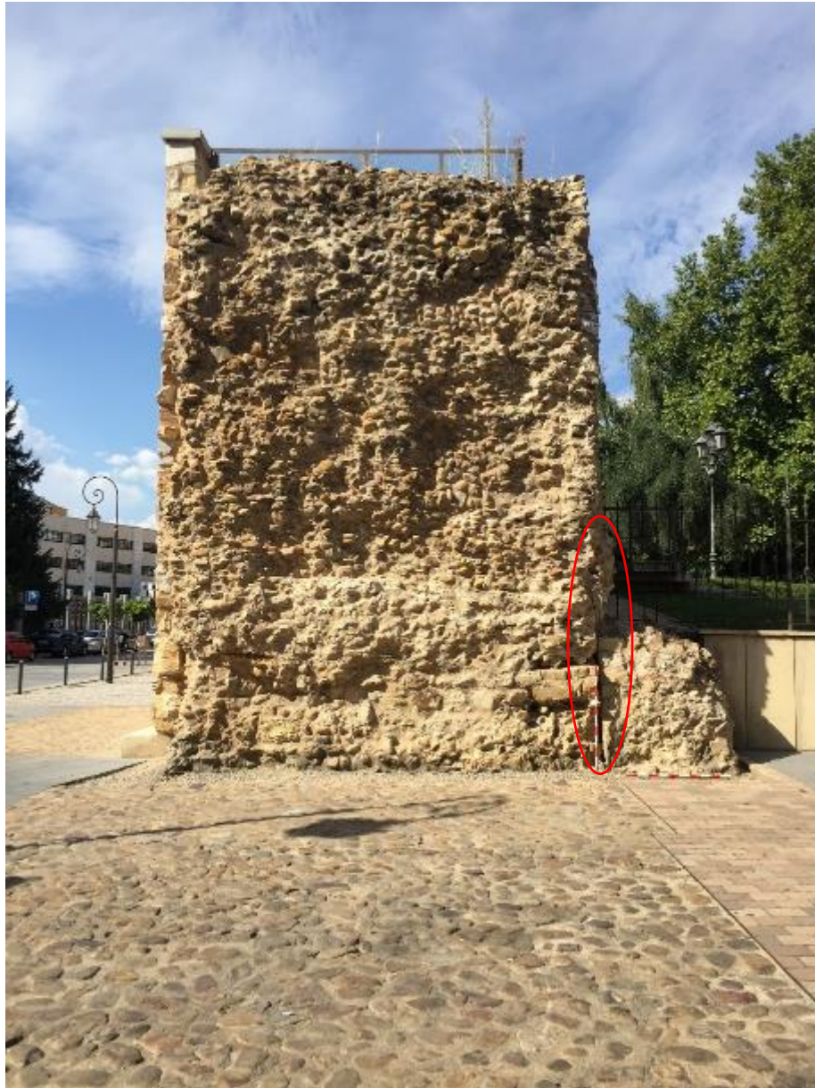
Fig. 78. Photograph of the two walls, the Early Imperial Roman one and the wall of cubos , in Calle Ruiz de Salazar, with the gap or breach between both of them. On the ground can be seen, via a floor layout of riverstones, the foundation of the missing section and the tower of the last Leonese wall of cubos , projected towards the outside of the walled enclosure in the lower right corner.
