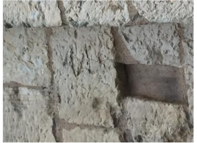
Fig. 9. Detailed photograph of ashlar with VI mark in situ on a blocked putlog hole. Tower of San Isidoro (León).
