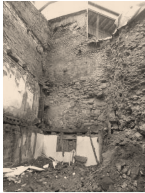
Figs. 108 and 109. State of the cubo at the southwest corner of the medieval wall after it collapsed in 2017: we can observe the filling layer of the cubo overlapping the medieval facing of the wall.
