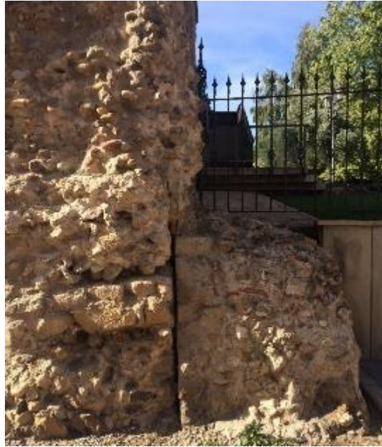
Fig. 111. Photograph of two walls attached, the cubos and the Roman wall, in Calle Ruiz de Salazar (in the background, the 'Romantic' or 'El Cid' park). The small-ashlar facing of the damaged Roman wall is covered by an overflow of lime and stone mortar from the wall of cubos that hardened over the fissure between the two walls.
