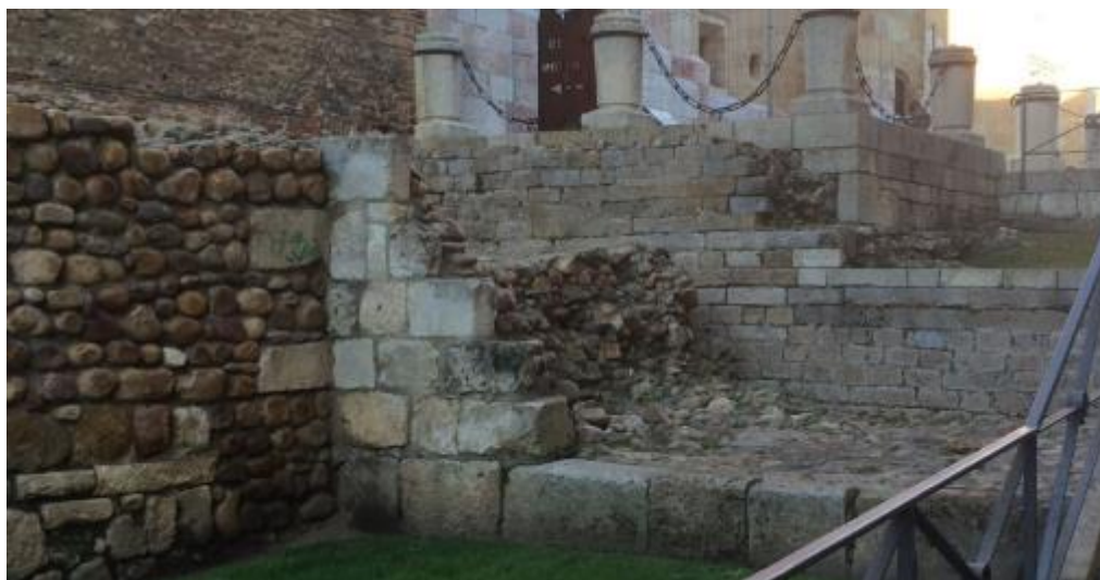
Fig. 54. In the background, the small-ashlar Roman wall, until now considered from the Flavian period (León III), to which the later wall “of cubos ” at the forefront is attached. A tower (or cubo ) is annexed to the wall of reused ashlars (access stairway to San Isidoro from Avda. Ramón y Cajal).
