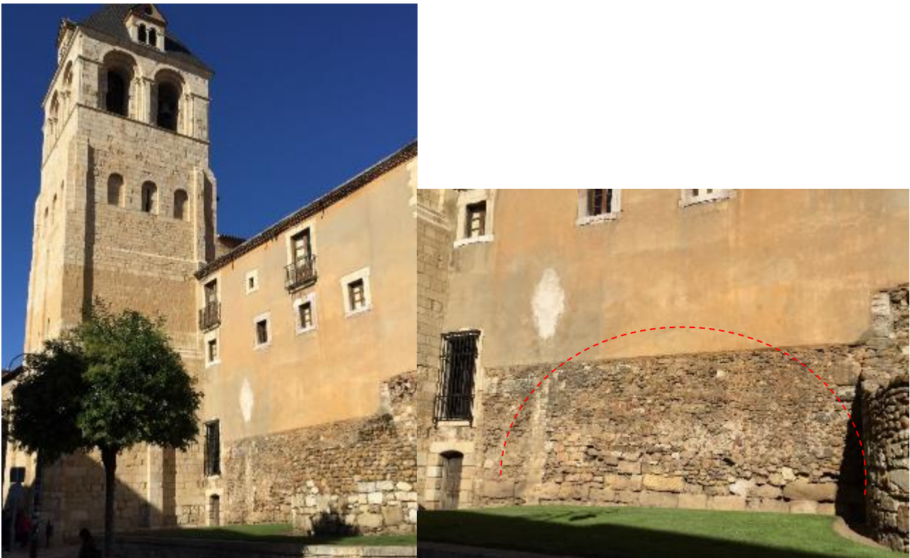
Figs. 61 and 62. Current photographs of the Torre del Gallo or San Isidoro Tower. To its right, you can see the blocked arch layout on the face of the wall of cubos .
