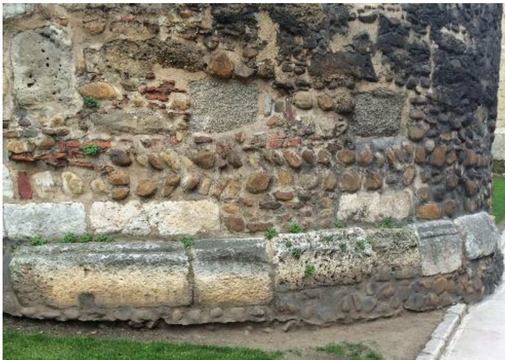
Fig. 103. Photograph of another tower ( cubo ) in the Avenida de Ramón y Cajal where moulding-finished ashlar are also reused in medieval masonry.
